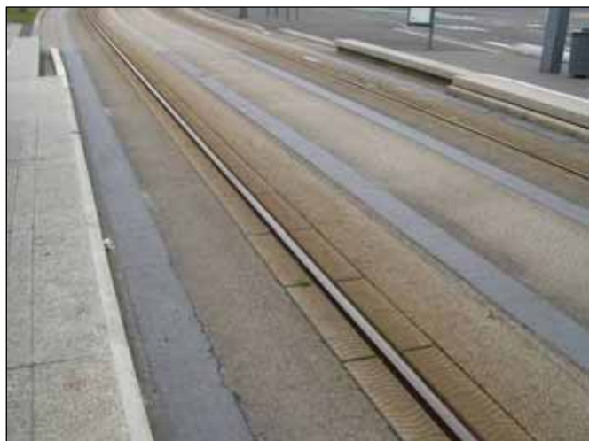
Figure 9: GLT central rail and concrete rutting repair
