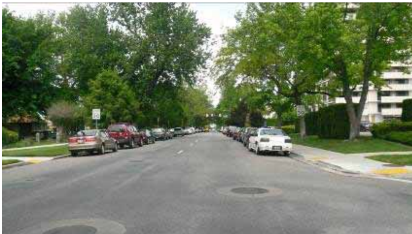
Idaho west of 2 nd approaching 3 rd ( westbound mixed traffic; parking remains )
