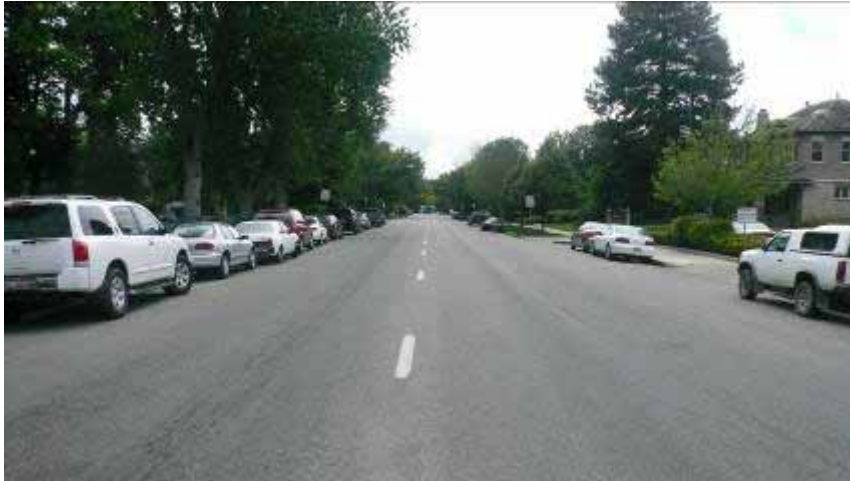
Main east of 3 rd approaching 2 nd ( eastbound mixed traffic; parking remains )
