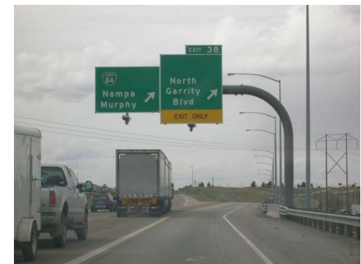
Garrity Blvd Double Lane Exit
