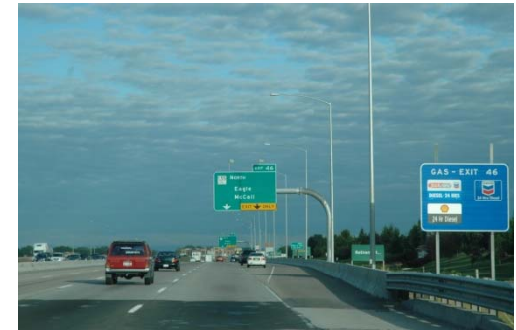
Eagle Road Double Lane Exit
