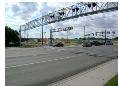
Eagle Road Un-Gated Crossing
