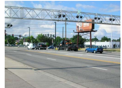
Cole Road Crossing Adjacent to Franklin Signal
