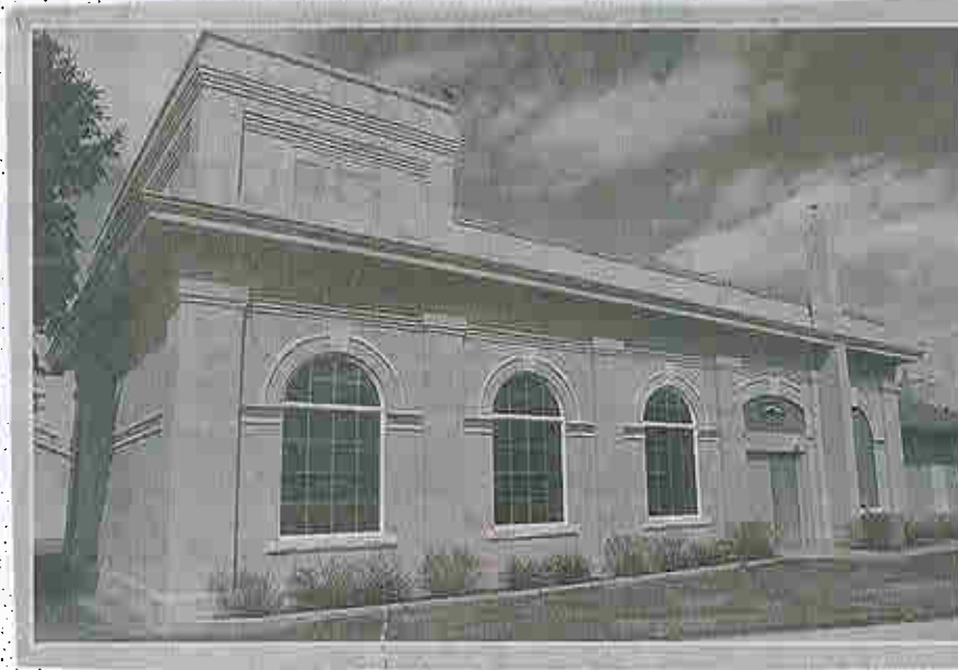
Trolley Station in Middleton is the former Idaho Power Substation, built about 1907 to power the Interurban streetcar line that made a loop around the Boise Valley. Nearby, but not pictured, is the original Interurban Station. The last car passed through Middleton en route to Caldwell at 6:04 p.m. May 17, 1928.
