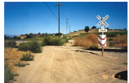
Figure 7 Unimproved Public Crossing with Crossbucks at Karcher Road
