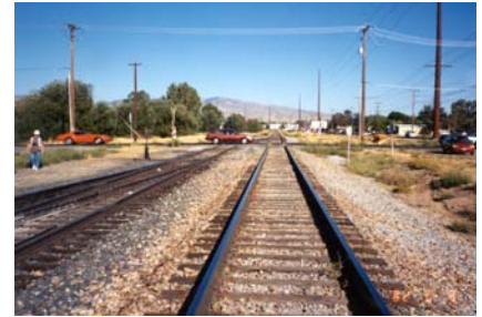
Figure 5 Typical Track with Siding
