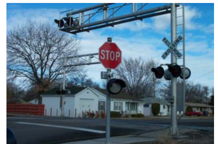
Figure 6 Crossing with Flashing Light and Crossbucks
